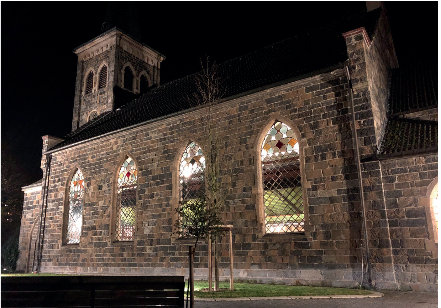
Church of the Redeemer, Schalksmühle, Germany. Luminaire: SILL 49M ©Hoffmeister
