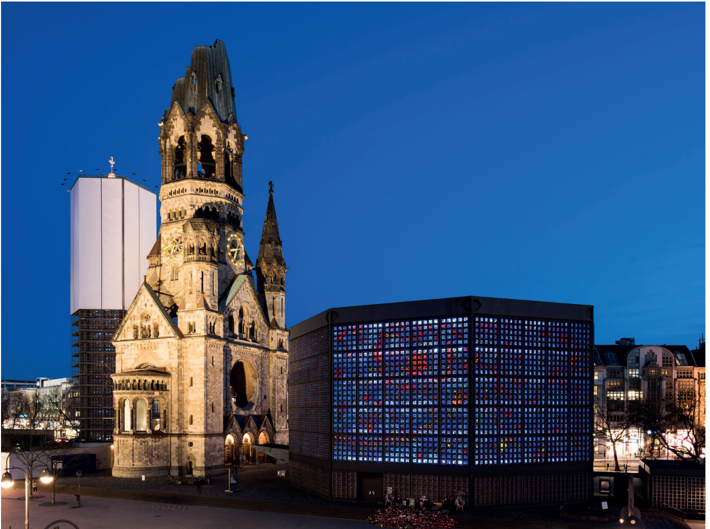
Kaiser Wilhelm Memorial Church, Berlin, Germany. Luminaire: 49. Light planning: Kardorff Ingenieure Lichtplanung GmbH ©Linus Lintner
